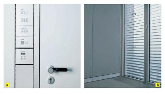
Fig. 8 The control panel next to office doors (a) and an interior view showing perforated aluminum blinds in the façade cavity (b) © Ingenhoven architects.
