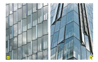
**Fig. 22** Façade detail showing flaps letting air into the façade cavity (a); flaps opened at the "tip" to enable through-flow of air (b)  $\bigcirc$  Jan Bitter.
