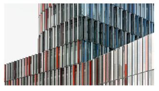
Fig. 17 Sawtooth profile façade with slender colored panels between larger fixed glass panels © Jan Bitter.
