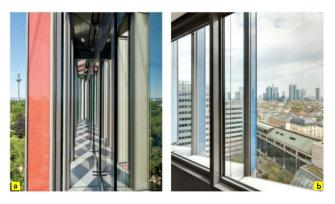
Fig. 18 View into the 700 mm continuous horizontal cavity of the double skin (a) © KfW-Bildarchiv/Thomas Klewar; Double-skin façade viewed from interior showing the colored glass panels that open by pivoting outwards (b) © Jan Bitter.
