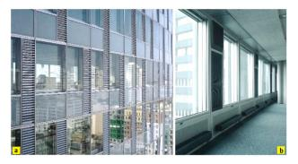
Fig. 11 Louvered air intake openings on the east façade (a); and the inner upper panels which pivot downward for air intake (b) © Annette Kisling.
